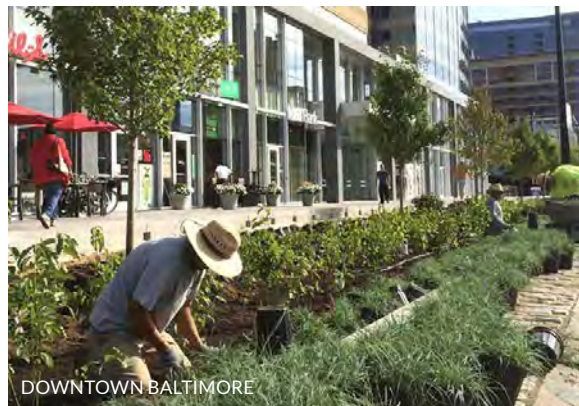
A bioswale along Pratt Street in downtown Baltimore helps filter pollution from rain water runoff before it drains into Baltimore Harbor.
